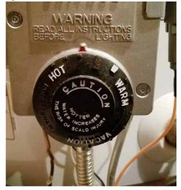
temperatures that are significantly different from the dial setting. A 10°F difference in outlet water temperature could make the difference between safe delivery of domestic hot water and the potential for a serious burn.
