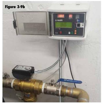
• Precise temperature control based on electronic temperature sensing at one or two locations in the system.
