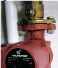
18. For circulators without internal check valves, the preferred mounting orientation is in a vertical pipe with upward flow. This allows air bubbles to naturally rise through the circulator's volute and out through the discharge port.
