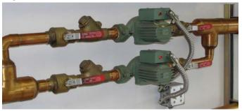
As is true with circulators in series, two identical circulators operating in parallel may reduce the circulator electrical power requirement compared to a single larger circulator that would yield the same flow rate in the circuit.
