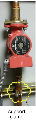
will require maintenance or replacement. This is simple and fast if there are ball valves, gate valves or butterfly valves on each side of the circulator that can be closed to isolate it from the balance of the system.
