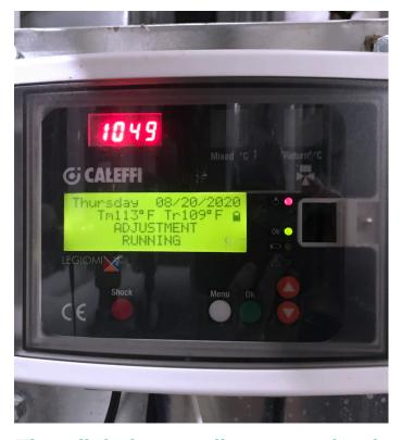
The digital recording capacity is comprehensive. All the parameters are updated daily and logged, with temperatures recorded every hour.
