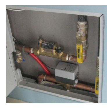
"It was so easy - we could have sent an apprentice to go around and accurately set the flows." Each room has an access panel with a QuickSetter balancing valve, used to properly balance the hot water circulating through the radiant tubing installed in the concrete floor. They were able to
