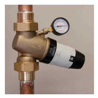
Lee likes the union connections of the PresCal valves, because he can mix and match connection types, depending on the project.
