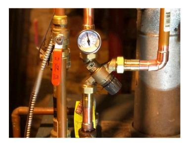
Maruffi installed a Caleffi AngleMix thermostatic mixing valve as a replacement. The angle shape of the body helped him work the valve into a tight space, without reworking a lot of the existing piping. He opted for the temperature gauge outlet to easily dial in the supply. "It was much easier than running up and down the stairs to check the mixed supply temperature," he said. The ball valves were able to be left fully open, as they were no longer needed now there was proper mixing.
