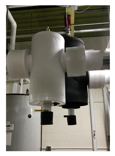
When challenged with a retrofit project, rescuing a system in need, Haan's ideal approach is to first flush and refill the system with the appropriate mixture of glycol and deionized water. Next, he likes to install an ECM circulator and protect it with a magnetic dirt filter. ECM circulators are an excellent way to reduce power consumption, but they need to be protected from magnetite and system debris.
