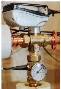
The initial scope of this Massachusetts school retrofit project was to replace aging thermostatic mixina valves that were in use for DHW. One of the three mixing assemblies scaled was and struggling to maintain a proper mixed water temperature. That wasn't going to cut it for the Facilities
