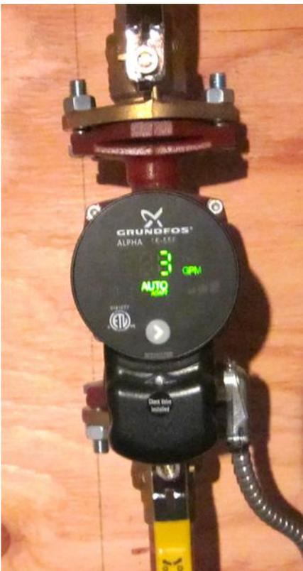
based on the circulator's power input, its RPM, and the internal calculation algorithms. They are capable of +/-5% accuracy when operated under the following conditions:
