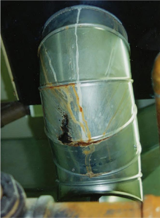
generally accepted guideline is to maintain the inlet water temperature to a boiler burning natural gas at or above 130°F.
