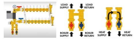
The H separator is used in applications to provide primary/secondary hydraulic separation at the mixing station. This application will require a primary pump pumping to the mixing station and will allow the pump in the mixing station to act as the secondary pump for the manifold.
