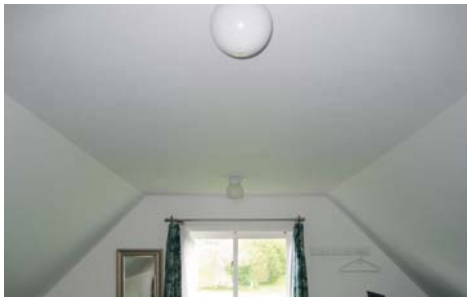
finished radiant wall
