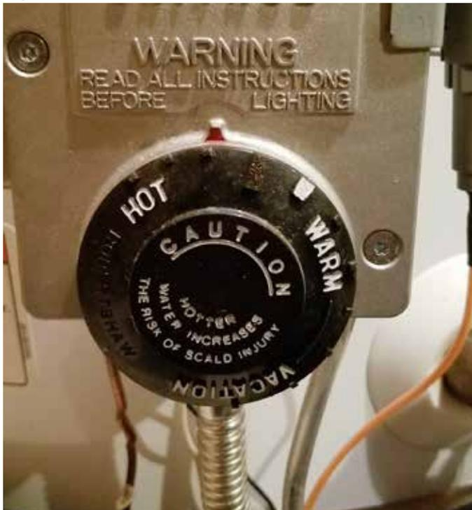
temperatures that are significantly different from the dial setting. A 10°F difference in outlet water temperature could make the difference between safe delivery of domestic hot water and the potential for a serious burn.
