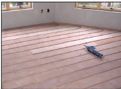
Photo of plywood sleepers glued and fastened to subfloor
