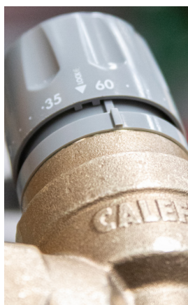
20 - Fit the new knob. The LOCK arrow should be slightly to the left of the reference notch
