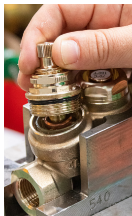
5 - Remove the headwork
