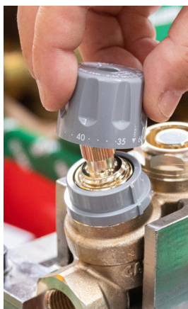
2 - Remove the knob (NOTE: keep the knob in a safe place)
