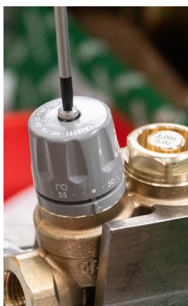
22 - Reposition at the desired setting value
