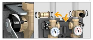
Installation differs depending on the supply direction in the flow circuit:
