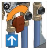
5. After carrying out these operations on all the outlets, it is possible to connect the electronic measurer to the sensor for the first branch and measure the corresponding flow rate. Flow rate regulation is performed by using the special knob to control the shut-off valve on the return manifold in correspondence with the same circuit, until the instrument indicates the design setting.
