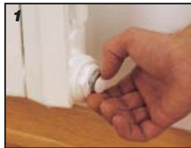
1 Remove protective cap
