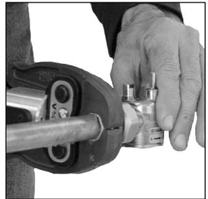
Check that the proper clamping jaws are installed and open jaw arms to set. Place jaw around valve end and double check proper insertion depth, press fitting.
