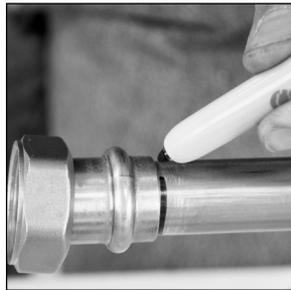
Insert the tube into the fitting, make sure the tube is fully inserted and mark with a marker to indicate proper insertion depth (7/8").
