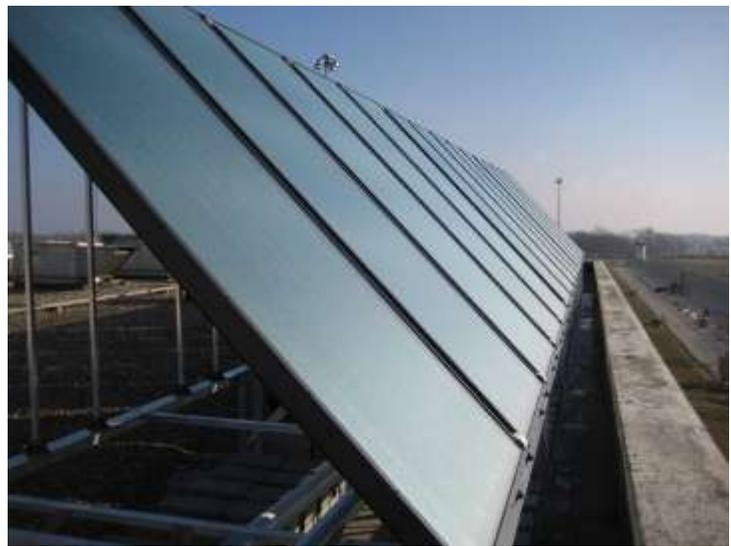
The Wabash Valley Correctional Facility is the first prison in the mid-west to utilize solar hot water to augment their heavy domestic water demands. Located in Carlisle, Indiana the facility installed a drain-back type solar hot water heating system early in 2011. The system is projected to save the prison about 40% of the cost to heat water amounting to \$6,000/year based on current fuel costs.
